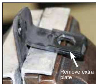
Photo 8 Before Plate Removal
