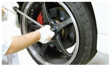
A floor jack was used to elevate the car and then it was placed on jack stands. Using an impact gun and the correct size socket the lug nuts were disconnected and the wheels and tires were removed.
