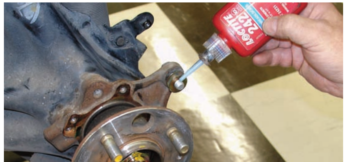
The bolts were coated with Loctite 271 before they were installed in the mounting bracket.
