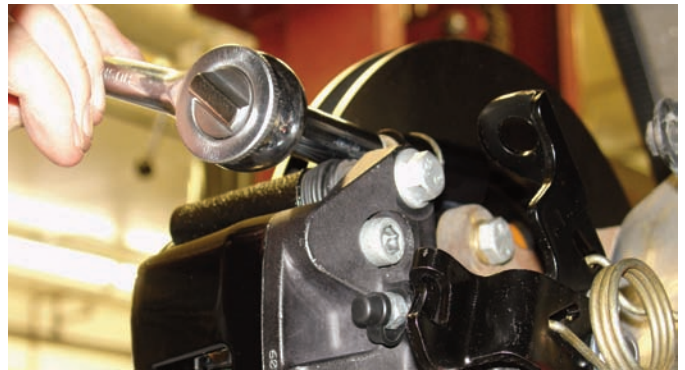
Using a socket wrench and the appropriate size socket the washers were installed followed by the self-locking nuts. They were tightened to 30 ft-lbs using a foot-pound torque wrench.
