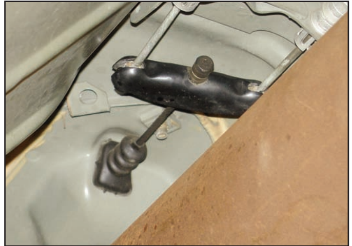
Photo 3. Installation of Cables to Balance Bar End
